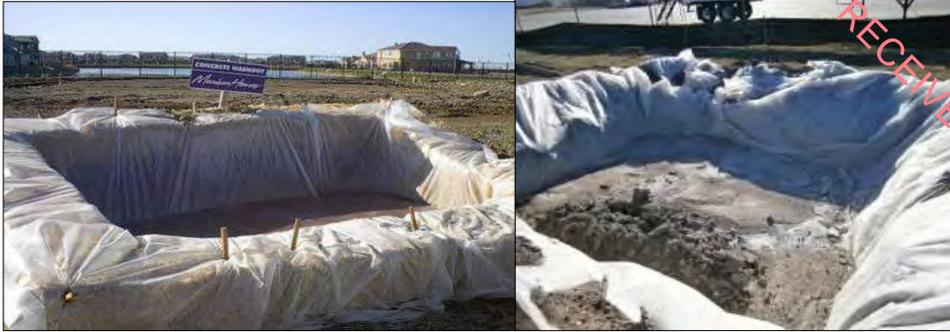
Plate 4-2 Concrete washout area
