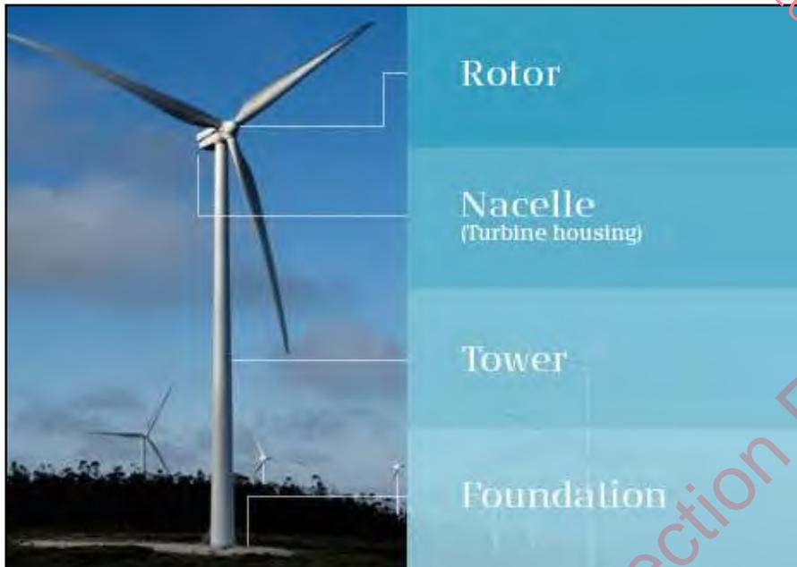
Plate 4-1 Wind turbine components
