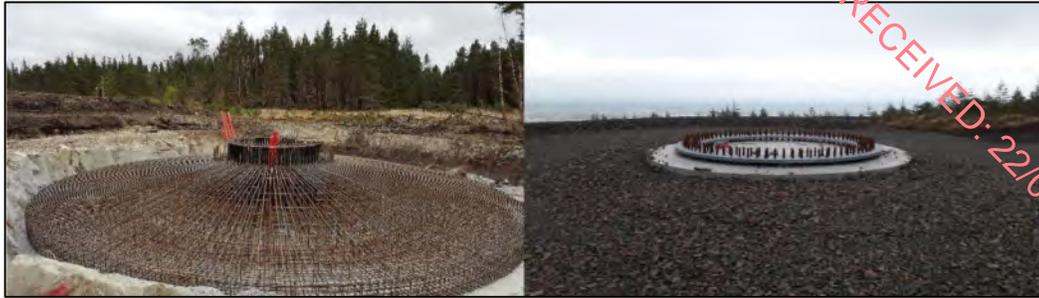
Plate 4-3 Turbine 'Anchor Cage' and finished turbine base
