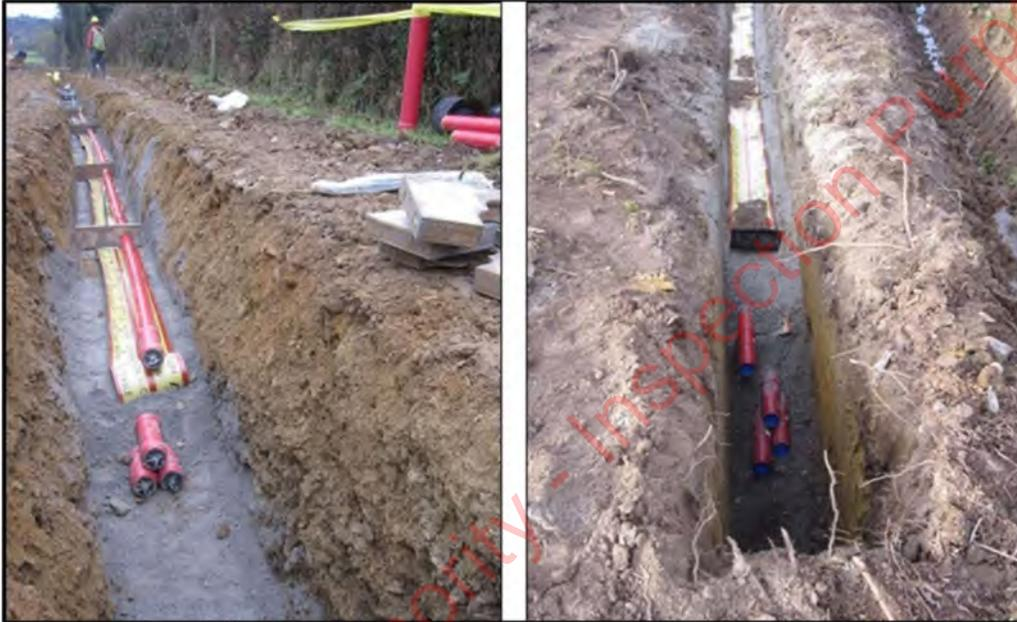
Plate 4-6 Standard Cable Trench View
