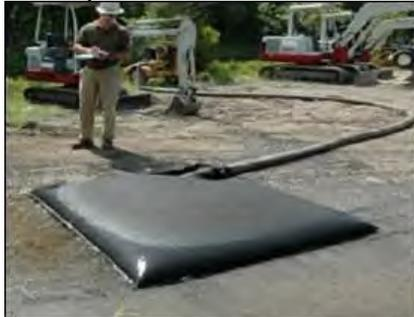
Plate 4-4 Silt Bag with water being pumped through
