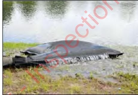
Plate 4-5 Silt bag under inspection
